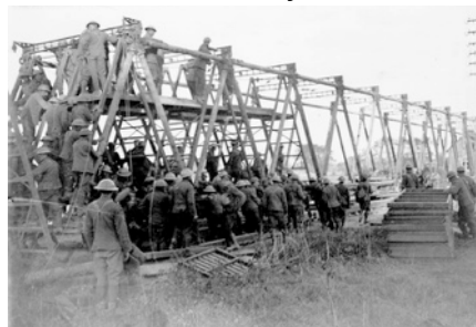
Canadian Combat Engineers building a bridge across the Canal du Nord
