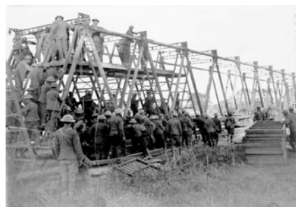
Canadian Combat Engineers building a bridge across the Canal du Nord
