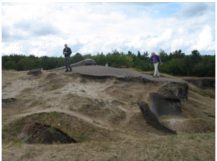
Fractured carapace on top of Fort Vaux
